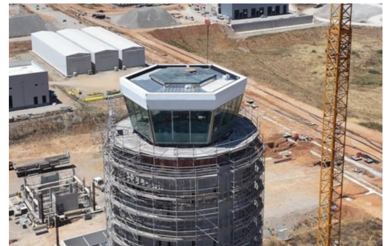
Control Tower Works
